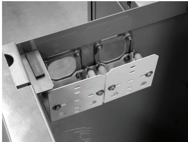
Figure 18. The mounting brackets for user-furnished fault indicators.
