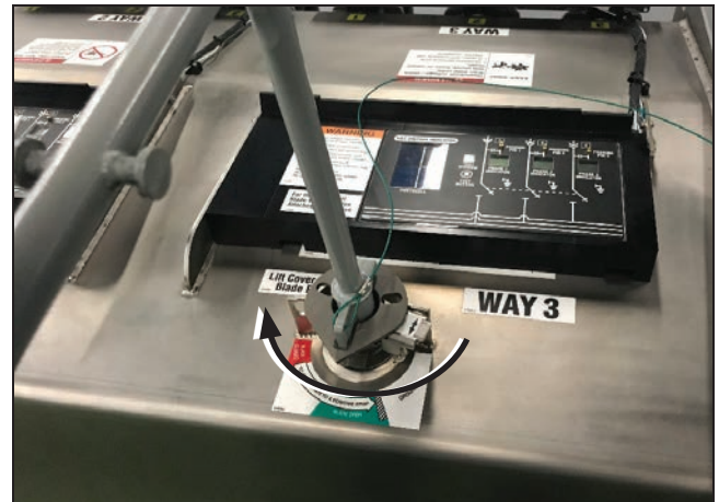
Figure 21. Closing the load-interrupter switch or fault interrupter.
