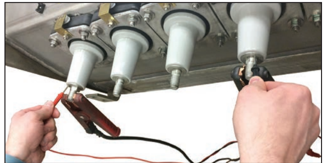
Figure 46. Connecting the resistance measuring device.●
