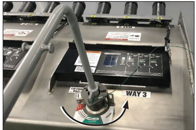
Figure 17. Operating from Open to Ground Position.
