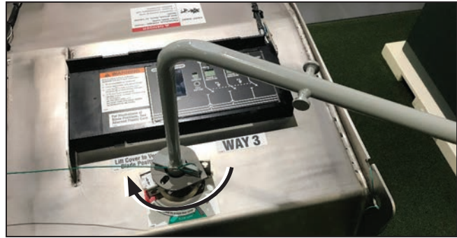
Figure 19. Operating from Grounded to Open position.
