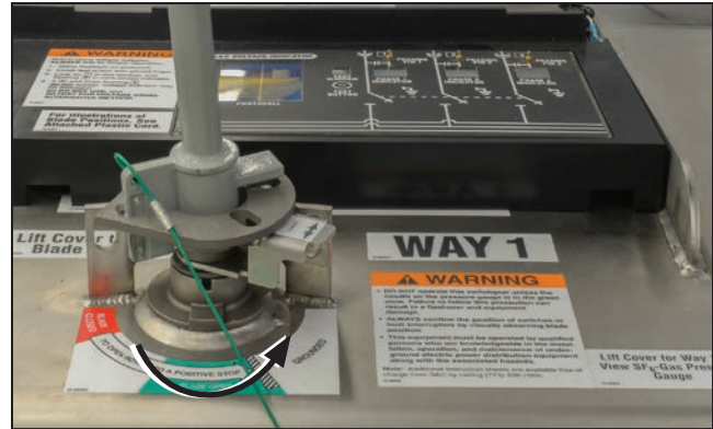
Figure 23. Rotate operating handle counterclockwise to the Open position.
