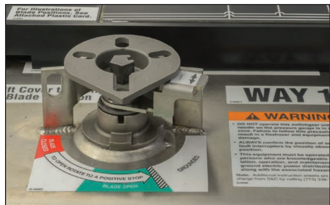
Figure 25. The fault interrupter in the Open position.
