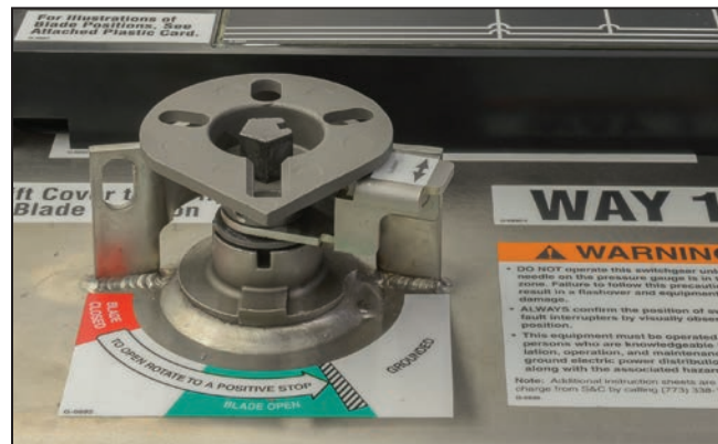
Figure 16. The load-interrupter switch or fault interrupter in the Open position.
