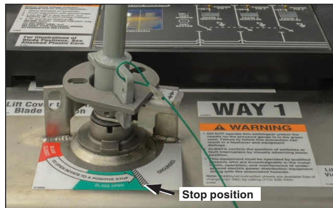
Figure 15. Rotate all the way to the Stop position.
