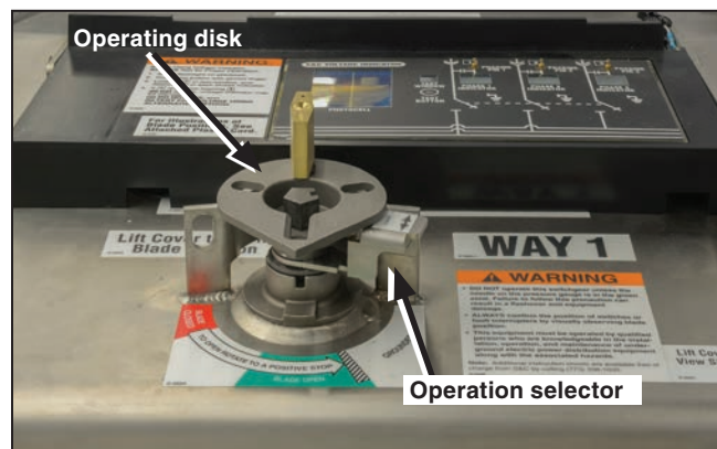
Figure 29. Locked in the Open position.
