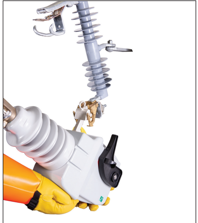
Figure 21. Lifting the trunnion out of the hinge of the cutout mounting using gloved hands.
