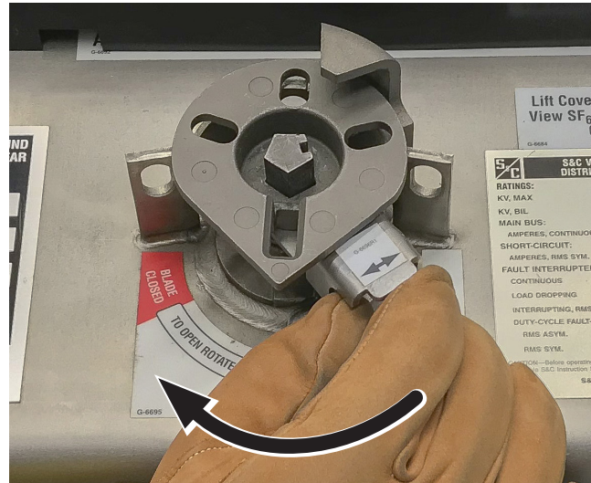
Figure 15. Rotating the operation selector to the far left enables operation to the Grounded position.
