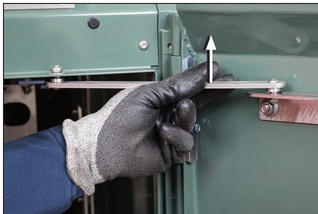
Figure 22. Lift the door-holder mechanism up to allow the door to swing closed.
