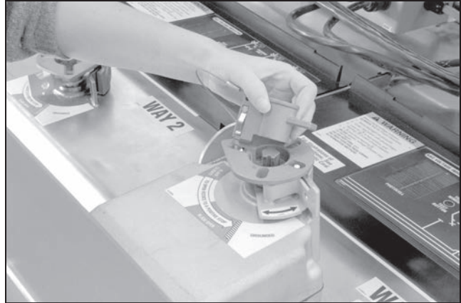
Figure 101. Remove the mechanical blocking key.
