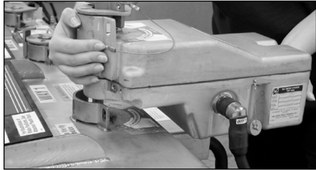
Figure 95. The motor operator placed over the operating shaft on the gear.
