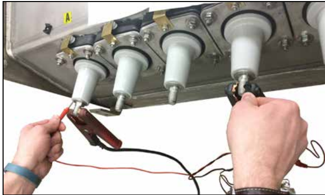
Figure 135. Connecting the resistance measuring device.●
