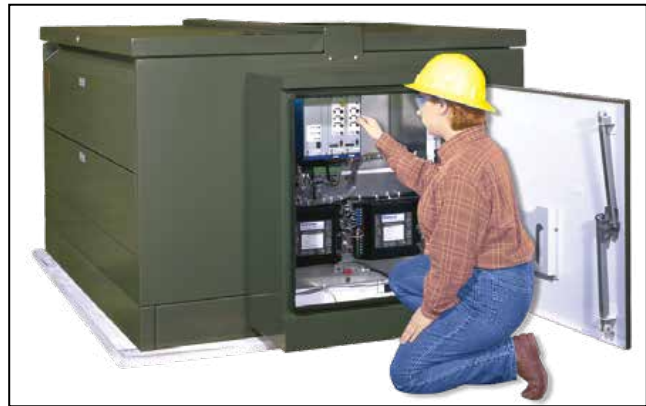
Figure 103. The location of the motor operator controls.
