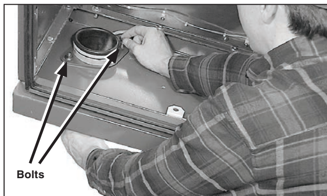
Figure 56. Install and secure the assembly through the wire pass.
