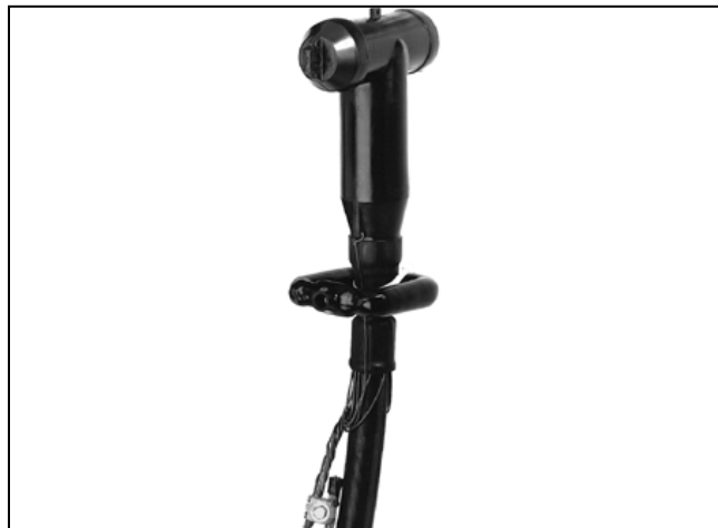
Figure 56. A current sensor placed above the cable's grounded concentric neutral.
