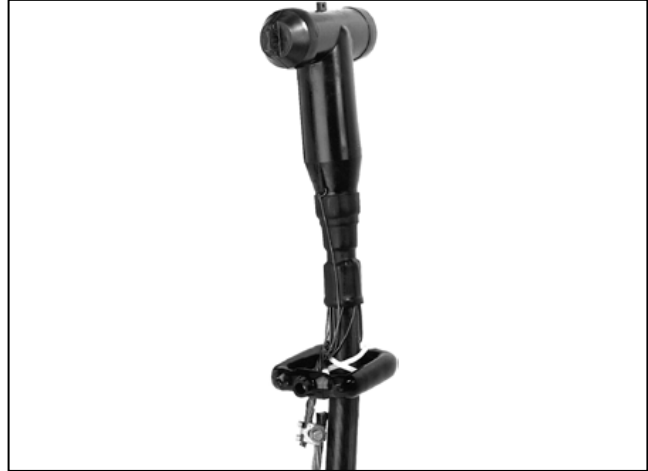
Figure 112. A current sensor placed around the cable’s grounded concentric neutral.●
