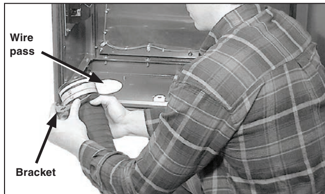
Figure 115. Place the holding brackets in the grooved channel of the conduit.
