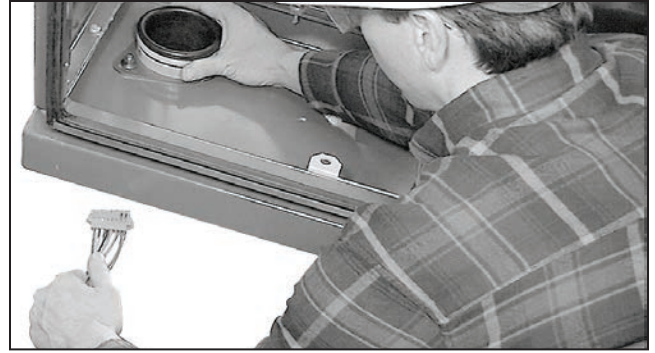
Figure 117. Channel the cables through the wire pass.
