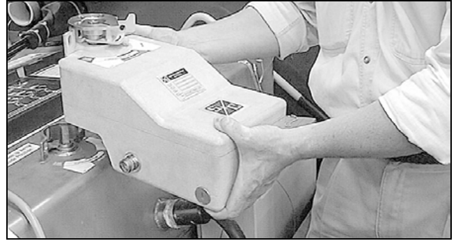
Figure 36. Placing the motor operator over the operating shaft on the gear.
