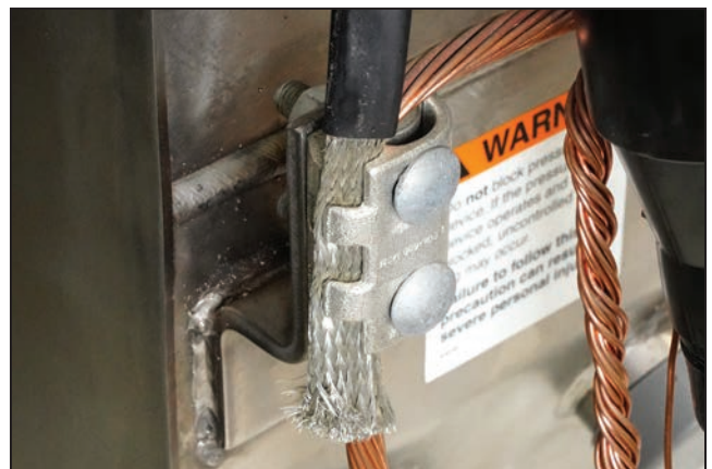
Figure 109. Connect shielded cable to tank ground.
