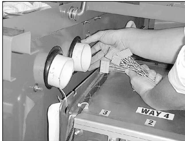
Figure 29. The cables being inserted through the PVC pipes.
