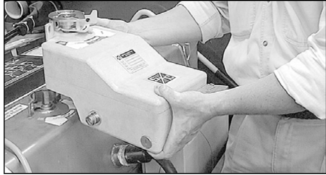
Figure 67. Placing the motor operator over the operating shaft on the gear.
