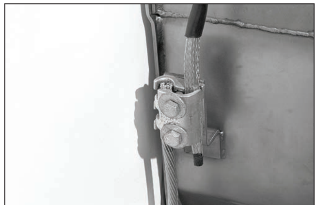
Figure 79. Connect the shielded cable to tank ground.
