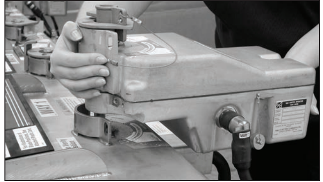
Figure 123. Place the motor operator over the operating shaft on the gear.
