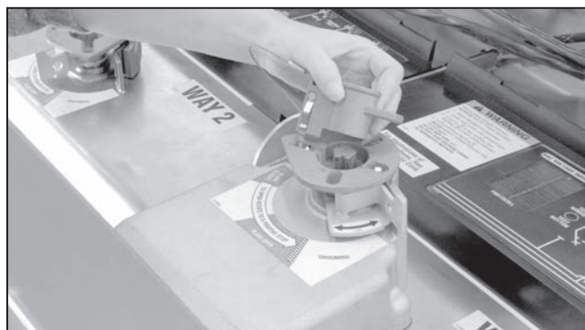
Figure 66. Insert the mechanical blocking key.
