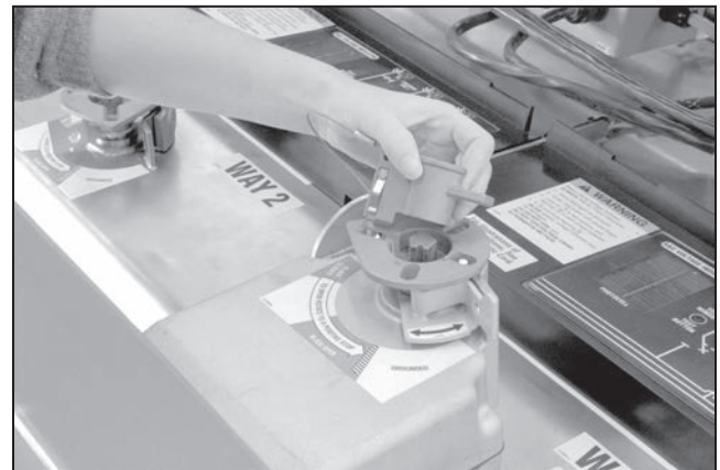
Figure 38. Remove the mechanical blocking key.
