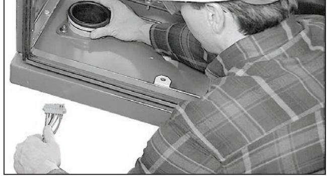
Figure 87. Channel the cables through the wire pass.
