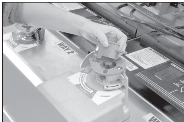
Figure 71. Remove the mechanical blocking key.
