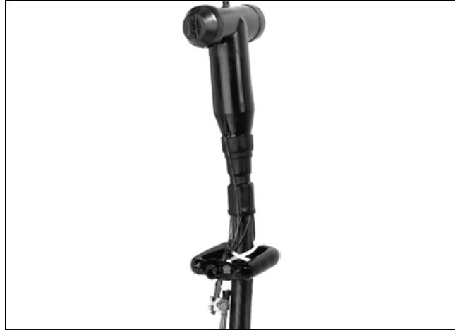
Figure 83. A current sensor placed around the cable's grounded concentric neutral.●
