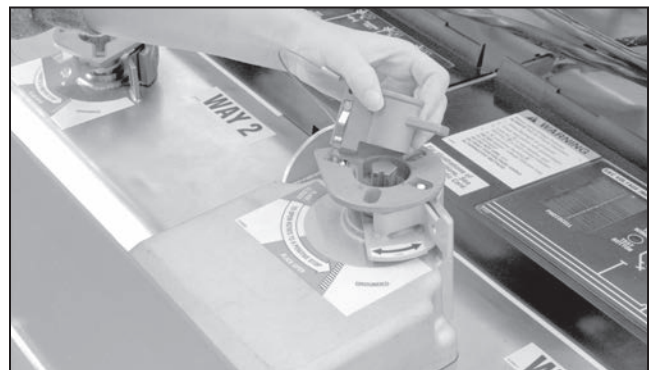
Figure 126. Insert the mechanical blocking key.
