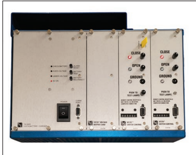
Figure 69. The Open indication on the motor control board matches the motor operator position.
