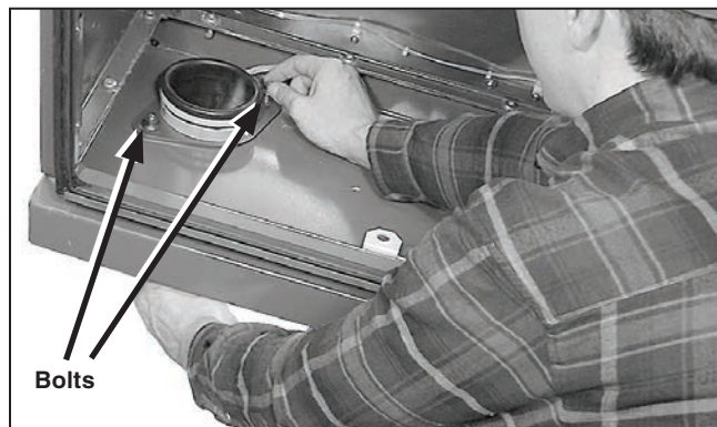
Figure 116. Install and secure the assembly through the wire pass.
