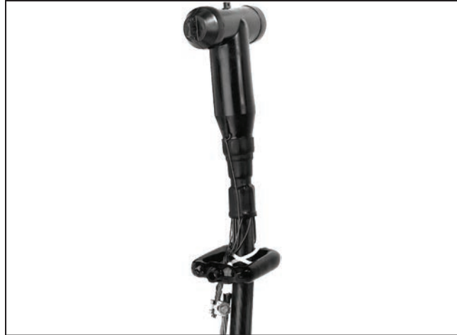
Figure 51. A current sensor placed around cable's grounded concentric neutral.
