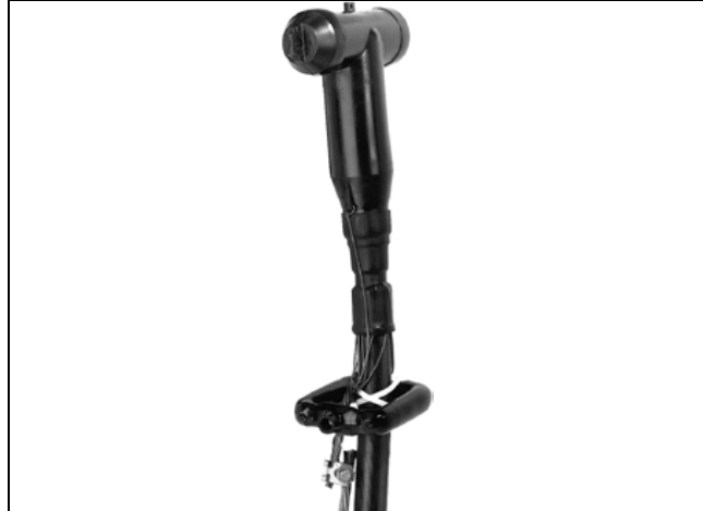
Figure 55. A current sensor placed around the cable's grounded concentric neutral.
