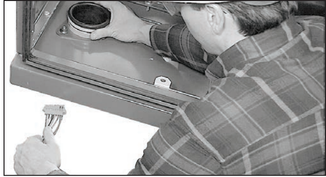
Figure 57. Channel cables through wire pass.
