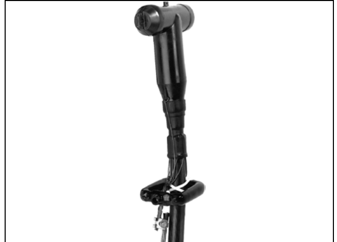
Figure 21. A current sensor placed around the cable’s grounded concentric neutral.
