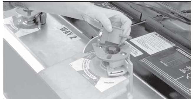
Figure 33. Insert the mechanical blocking key.
