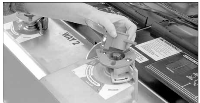
Figure 105. The mechanical blocking key.
