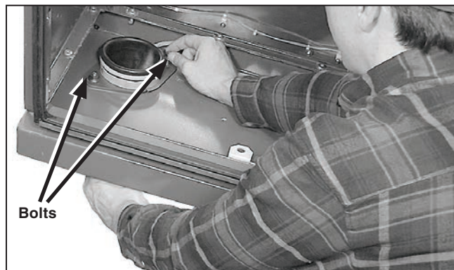
Figure 86. Install and secure the assembly through the wire pass.
