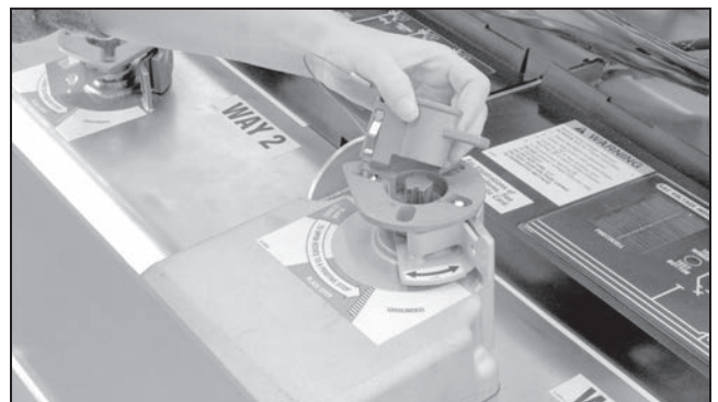
Figure 96. Insert the mechanical blocking key.
