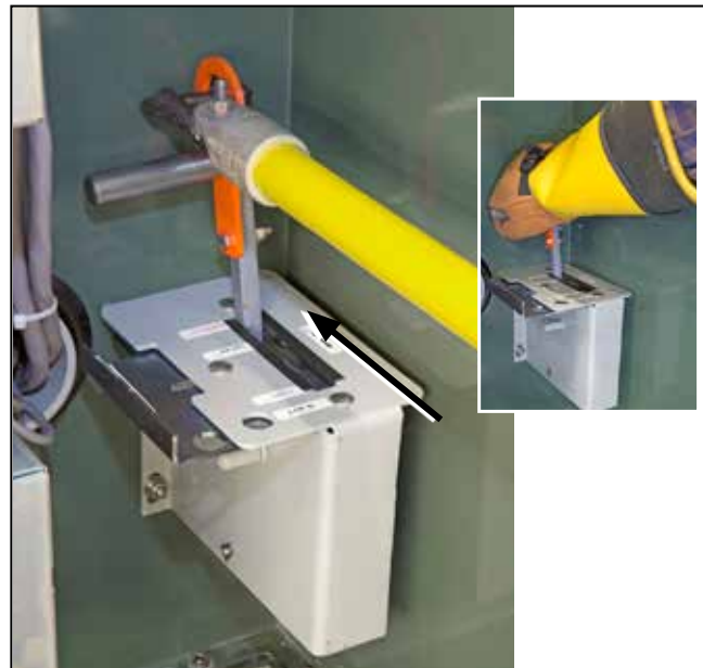
Figure 14. To close the interrupters, remove the tag (if present) and slide the interlock bar to the left to middle position. Push the OPEN/CLOSE/READY lever to Ready position. Slide the interlock bar to the left-most position, and push the OPEN/CLOSE/READY lever once to effect the first closing profile or twice, without delay, to effect the second closing profile.
