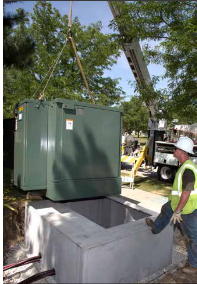
Figure 1. Lifting the Pad-Mounted Style IntelliRupter fault interrupter.
