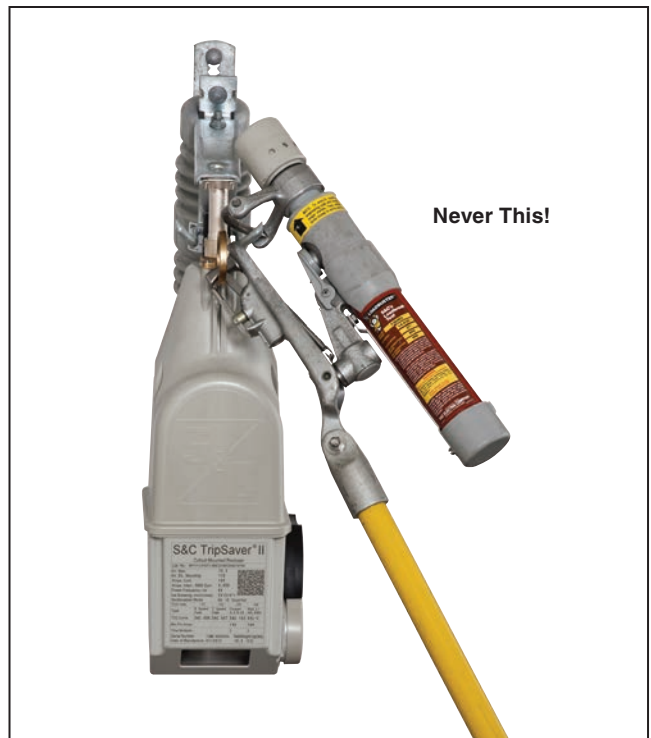
Figure 30. An incorrect fastening approach.
