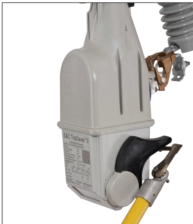
Figure 17. The curved label must be completely covered.
