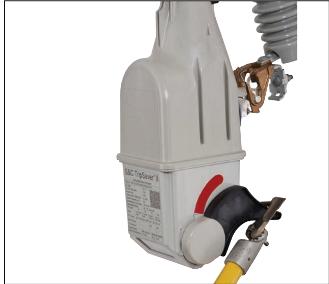
Figure 15a. A TripSaver II recloser entering NR mode.
