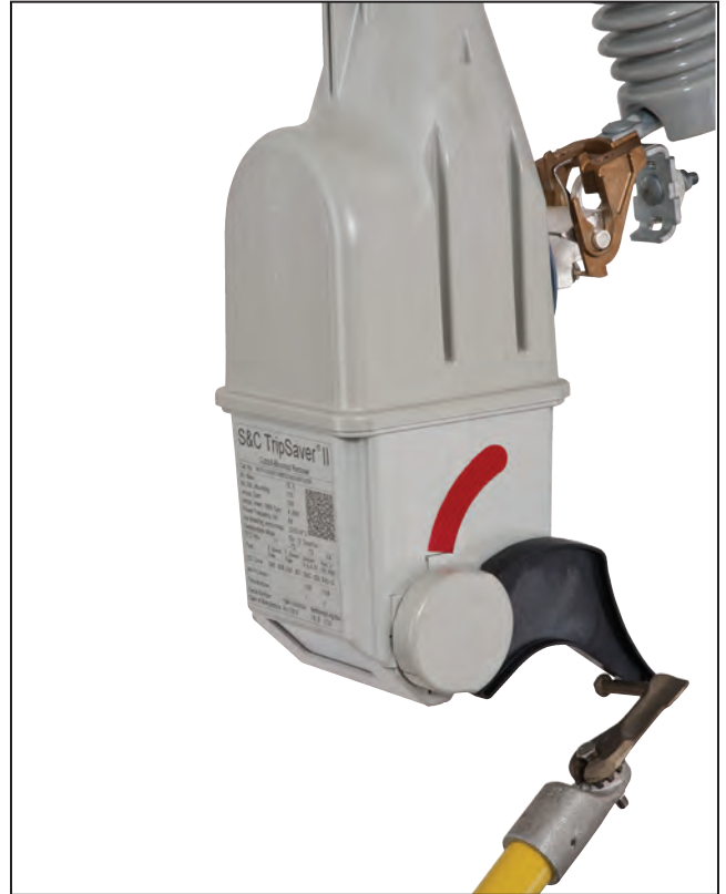
Figure 22. Place the prong under the lever and push it up.
