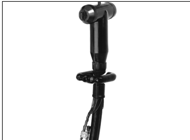
Figure 115. A current sensor placed above the cable’s grounded concentric neutral.●
