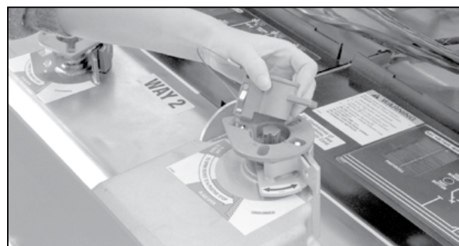
Figure 77. The mechanical blocking key.
