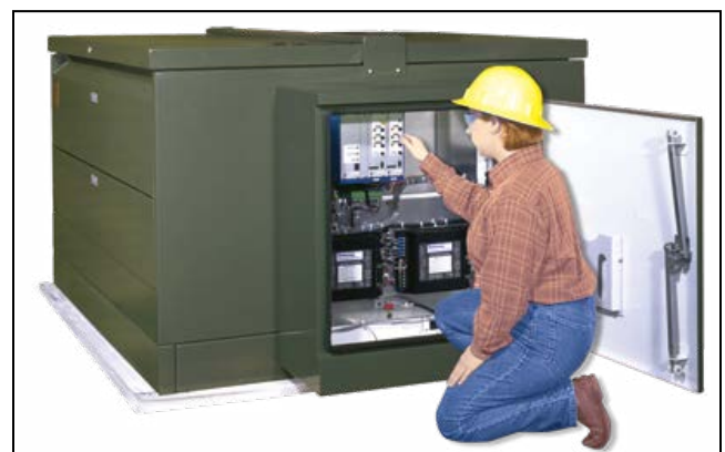
Figure 105. The location of the motor operator controls.
