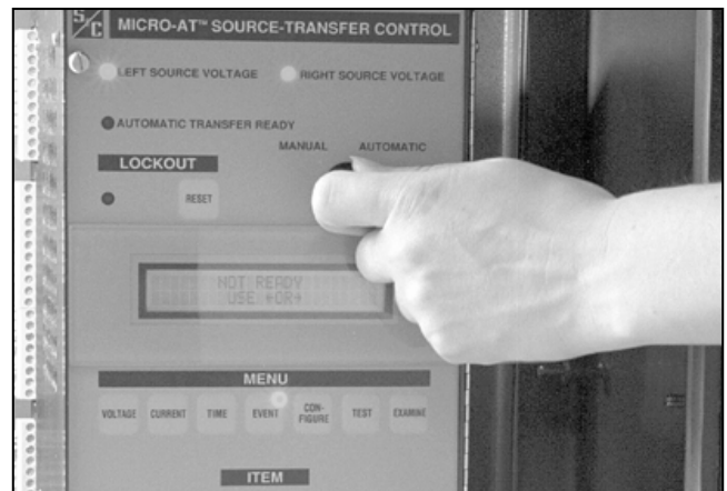
Figure 104. The MANUAL/AUTOMATIC switch on the Micro-AT Source-Transfer Control.
