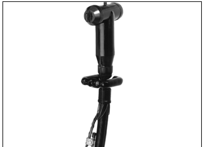
Figure 22. A current sensor placed above the cable’s grounded concentric neutral.
