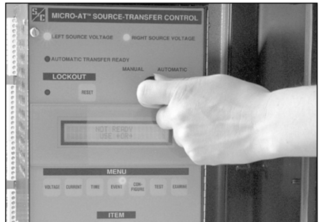
Figure 44. The MANUAL/AUTOMATIC switch on the Micro-AT Source-Transfer Control.
