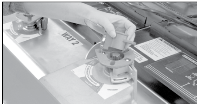
Figure 71. The mechanical blocking key.
