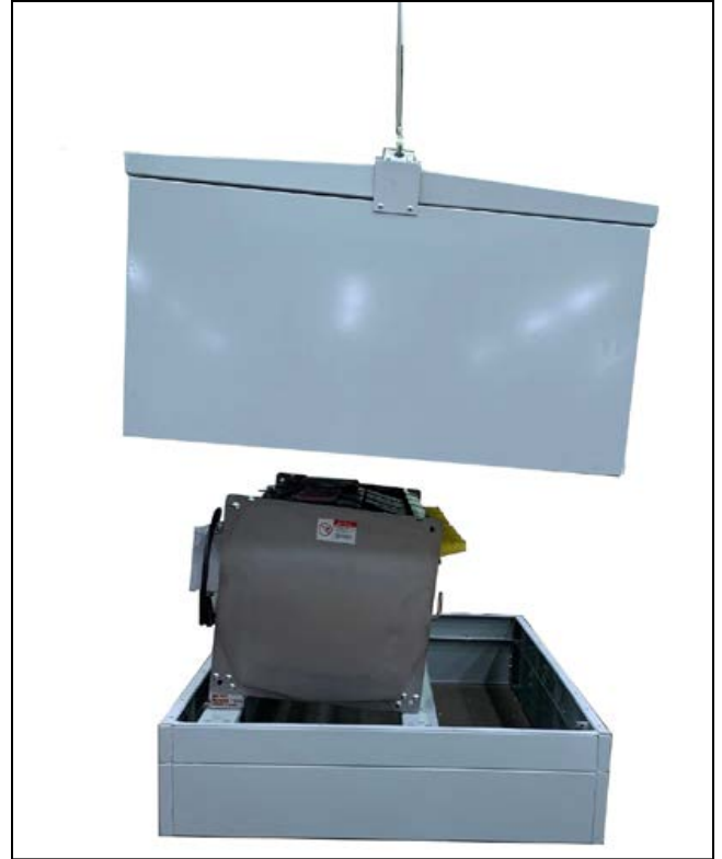
Figure 12. A pad-mounted style high-voltage enclosure being removed from the base spacer.
