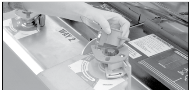
Figure 129. The mechanical blocking key.
