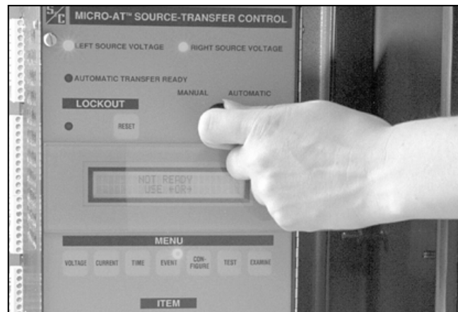
Figure 134. The MANUAL/AUTOMATIC switch on the Micro-AT Source-Transfer Control.
