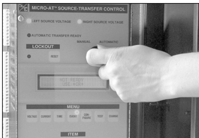
Figure 74. The MANUAL/AUTOMATIC switch on the Micro-AT Source-Transfer Control.
