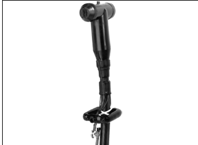
Figure 114. A current sensor placed around the cable’s grounded concentric neutral.●
