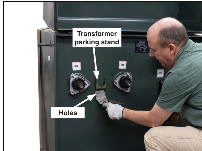
Figure 10. Slide the parking stand link bracket in from the bottom.
