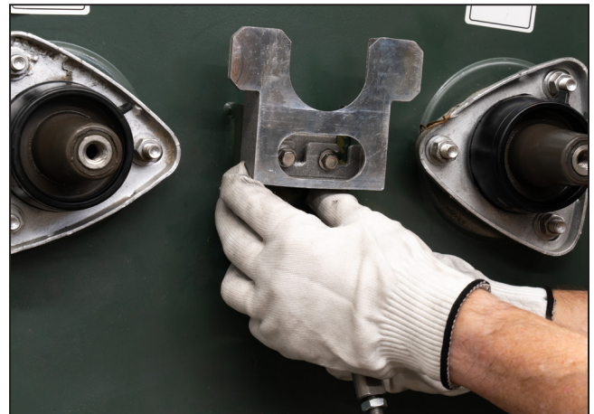
Figure 14. Slide the bolts into the grooves. Pull back on the bracket to hold the bolts against the parking stand radius.
