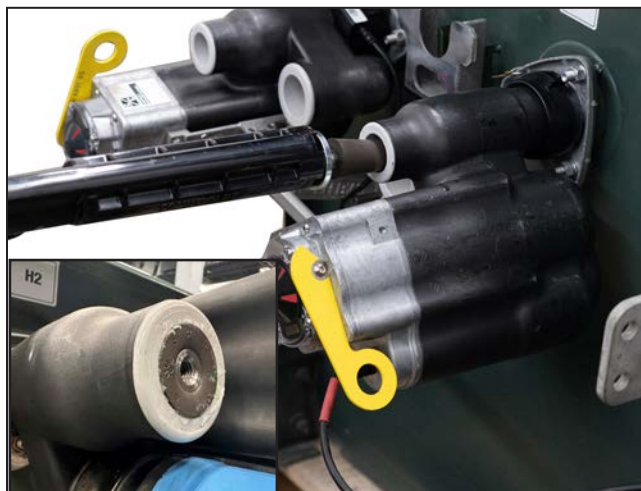
Figure 40. Push into the bushing well interrupter until flush with the bushing well interrupter opening.
