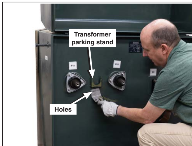
Figure 10. Slide the parking stand link bracket in from the bottom.
