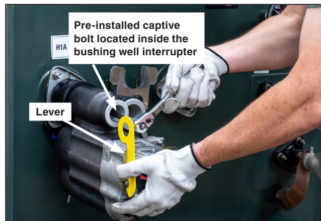
Figure 20. Align the bushing well interrupter with the bushing well insert. Torque the captive bolt.
