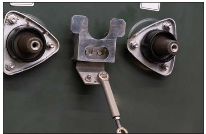
Figure 16. A completed parking stand link bracket installation.
