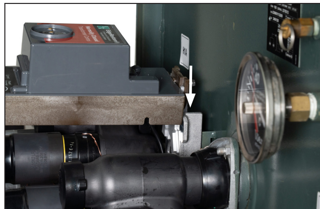
Figure 38. Control is slid onto parking stand.
