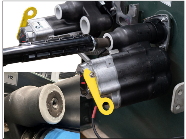
Figure 30. Push into the bushing well interrupter until flush with the bushing well interrupter opening.
