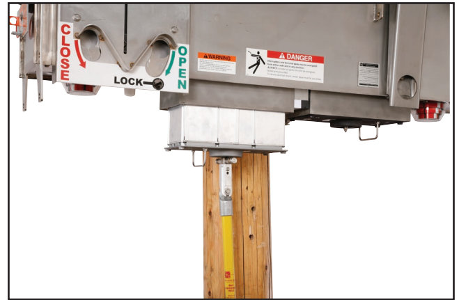
Figure 2. Removing the communication module from the base.
