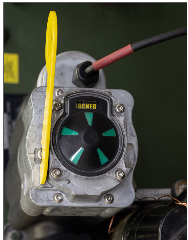
Figure 12. The bushing well interrupter in the Open and Locked position.
