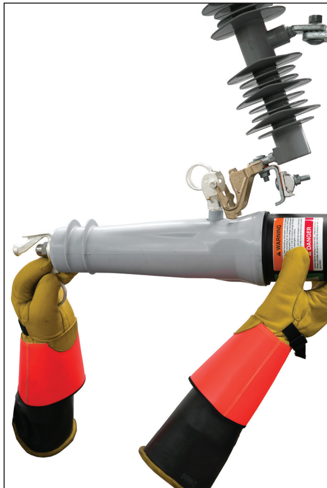
Figure 14. Removing the VacuFuse II interrupter with gloved hands.
