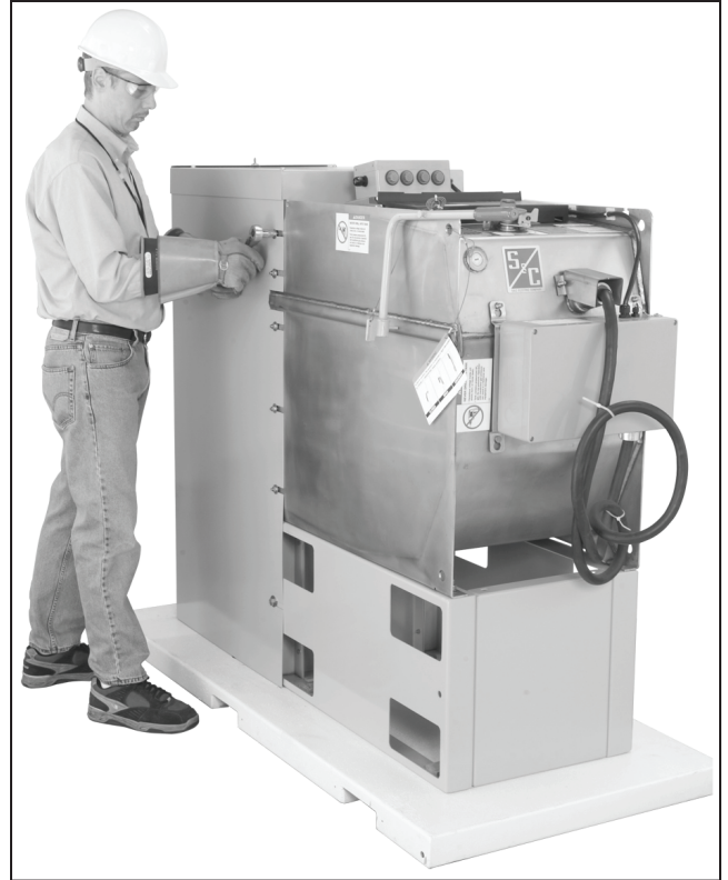
Figure 8. Tighten the six hex nuts retained on the studs.
