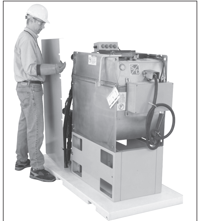
Figure 2. Remove the right side cover by pulling it forward.
