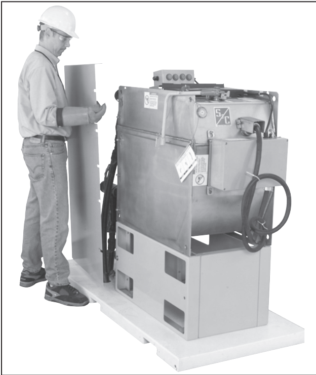
Figure 6. Slide the right side cover over the six studs.
