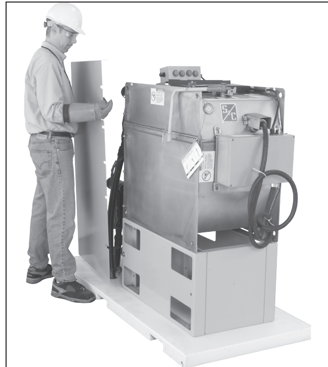
Figure 7. Slide the right side cover over the six studs.
