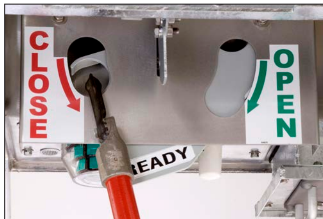
Figure 27. Closing interrupters with a hookstick.
