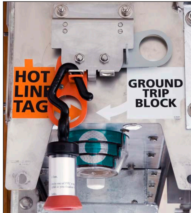
Figure 29. Hot line tag manually applied and “tagged.”
