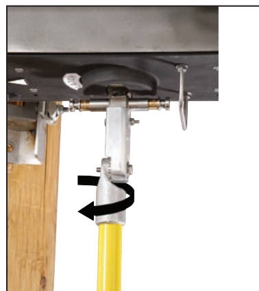
Figure 18. Locking the module into the base.
