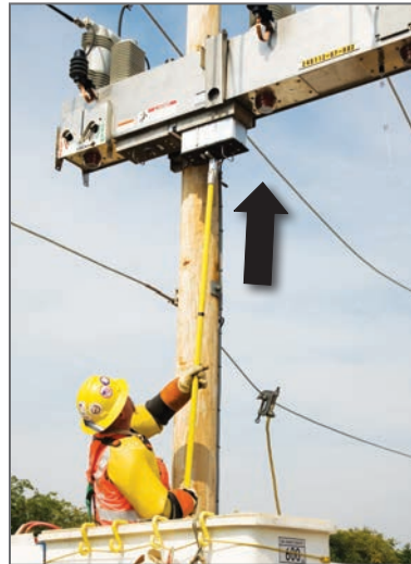
Figure 17. Inserting the module into the bay in the base.
