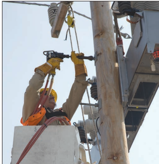
Figure 9. Tightening the through-bolts. Make sure a flat washer is between the bolt head and the mounting bracket.
