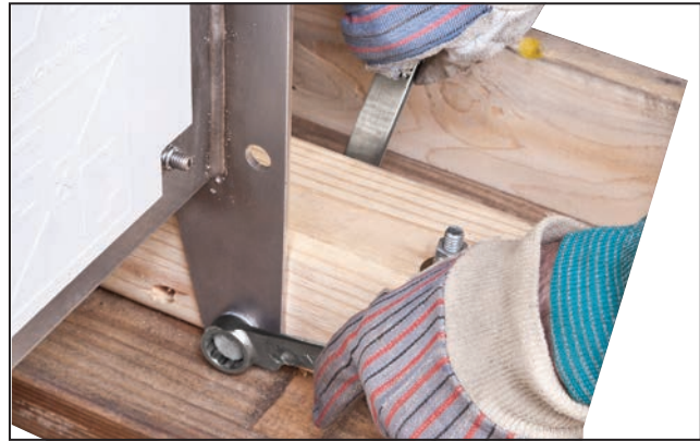
Figure 3. Unbolting a fault interrupter from the shipping supports.
