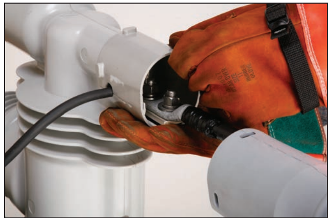
Figure 11. Installing the upper terminal-pad cover.
