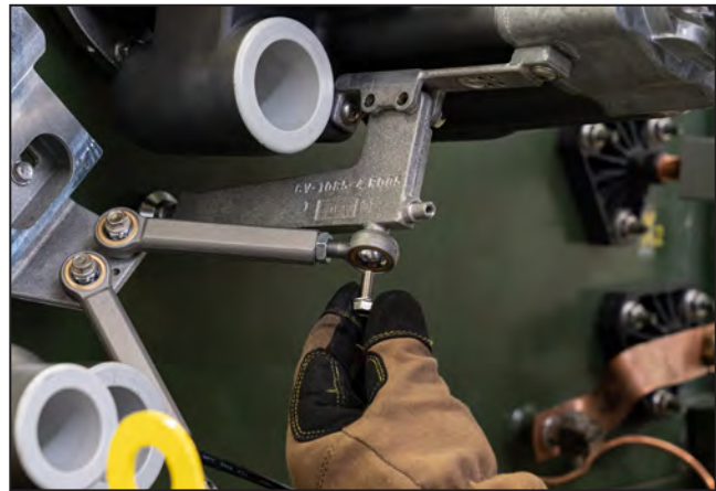
Figure 21. Install a bolt to connect the adjustable link to the swivel foot bracket.
