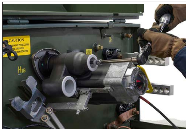
Figure 19. H1B bushing well interrupter installation.
