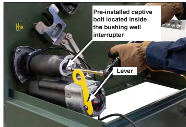
Figure 18. Align the bushing well interrupter with the bushing well insert. Torque the captive bolt.
