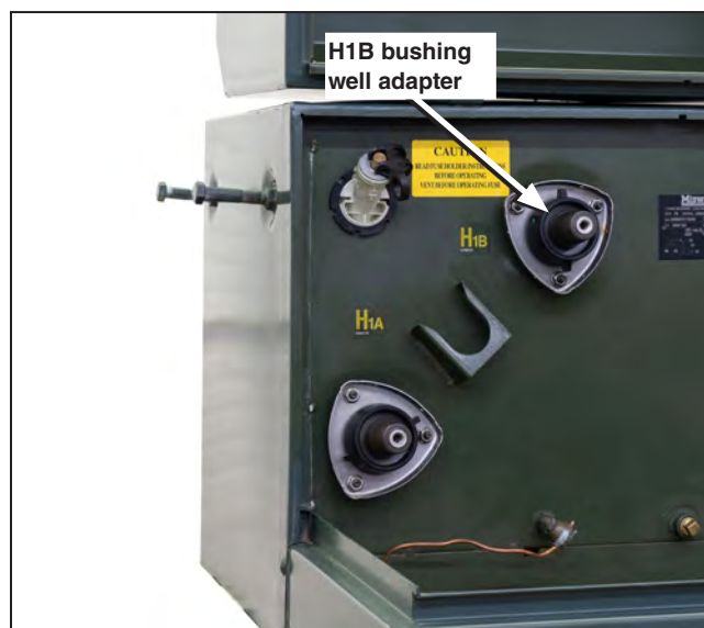
Figure 7. Installed bushing well adapters.
