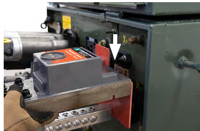
Figure 38. Hang the control on the hanger.
