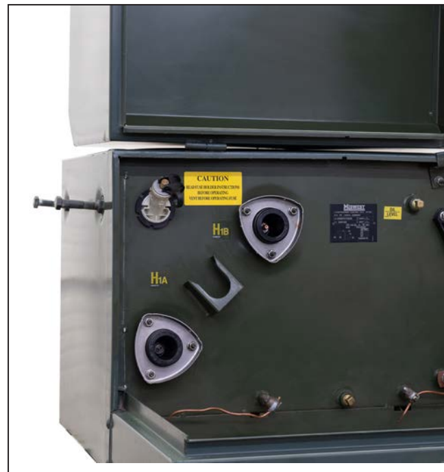
Figure 5. Bushing wells with loadbreak inserts removed.
