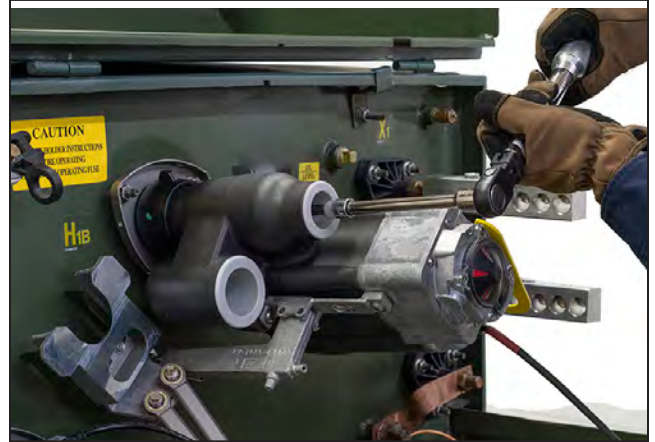
Figure 19. H1B bushing well interrupter installation.
