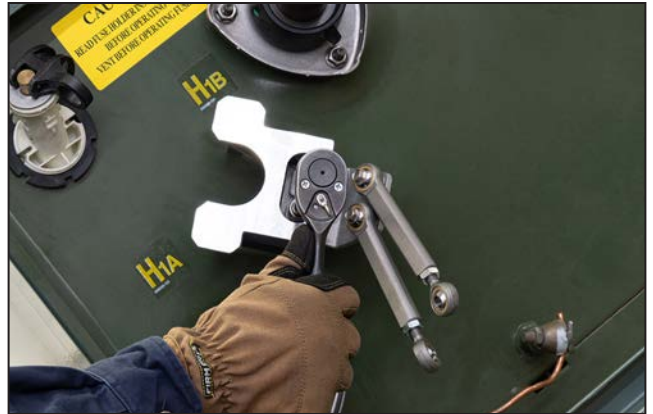
Figure 15. Tighten the bolts.
