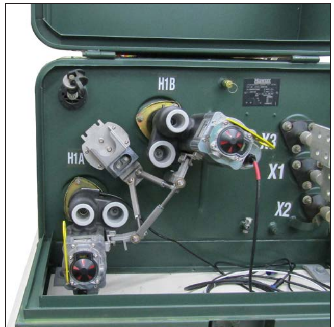
Figure 31. A completed parking stand spacer installation.
