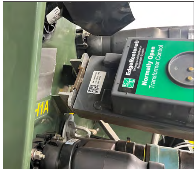
Figure 40. Hanging the control on the parking stand.
