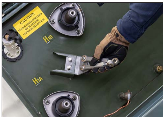
Figure 12. Pull down until the bolts hit the radius of the stand's opening.
