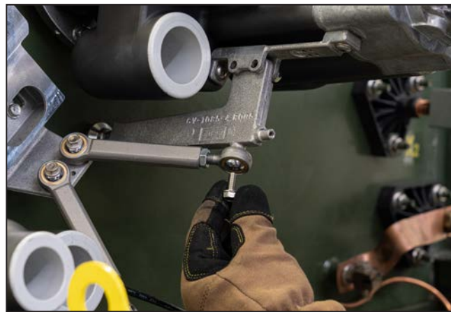
Figure 21. Install a bolt to connect the adjustable link to the swivel foot bracket.
