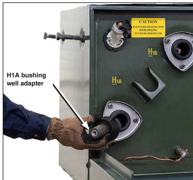
Figure 6. Before installing the bushing well adapter, grease the taper to be inserted.
