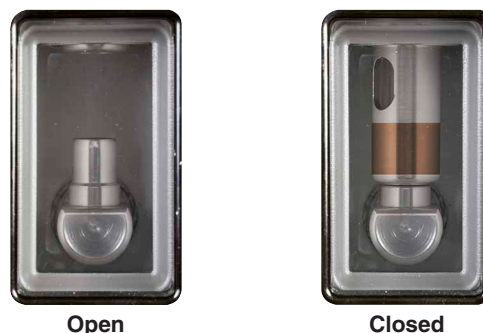
Figure 17. The visible-open gap (isolating disconnect) is easy to see through large viewing windows.
