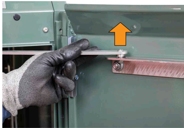
Figure 18. Lift the door-holder mechanism up to allow the door to swing closed.
