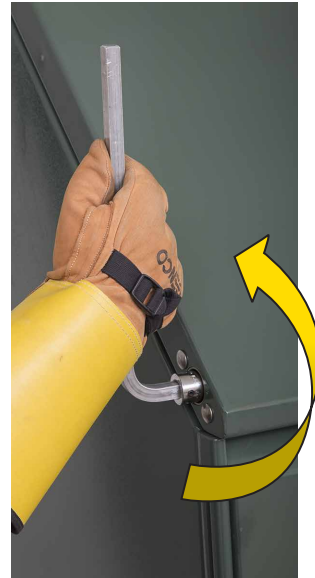
Figure 10. Unlatching the pentahead bolt latching mechanism with a pentahead socket wrench—a 360° counterclockwise turn will unlock the hinged roof.
