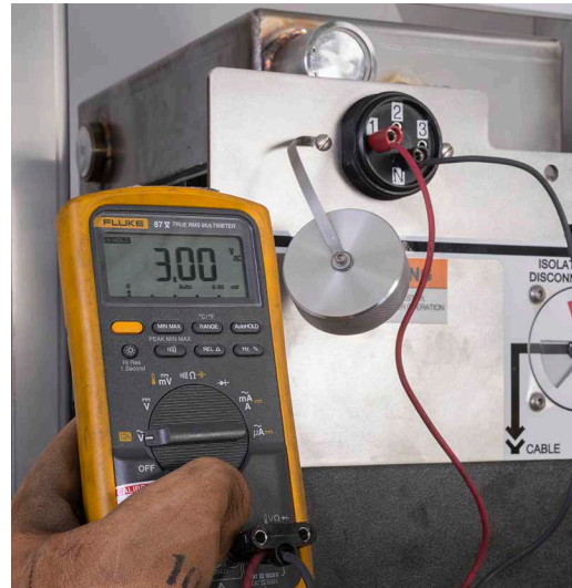
Figure 30. Check for voltage.
