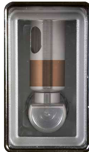
Figure 27. The isolating disconnect after the fault interrupter has been closed.
