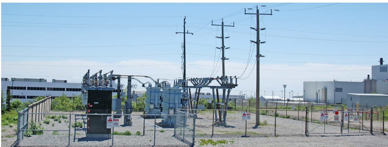
Open-air substation. Footprint: 50' × 50' (15 m × 15 m). Requires safety fence and ground grid.
