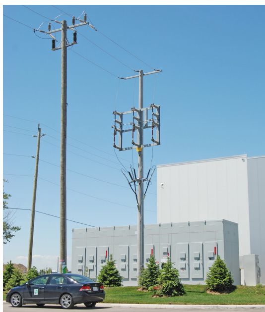
Open-air substation. Footprint: 50' × 50' (15 m × 15 m). Requires safety fence and ground grid.
