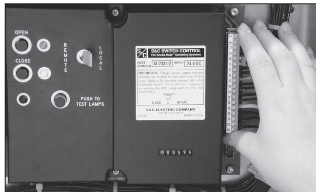
Figure 15. Remove the 18-pin terminal strip
