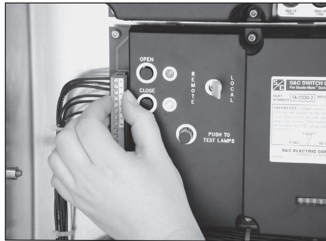
Figure 14. Remove the 12-pin terminal strip.
