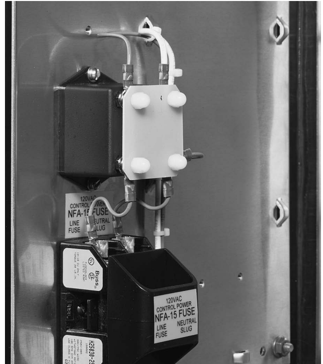
Figure 13. Connect external ac control power to the fuse block.
