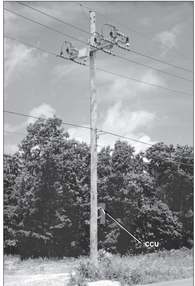
Figure 5. To minimize exposure to vandals the communication and control unit should be mounted at least 10 feet (305 cm) above ground level.
