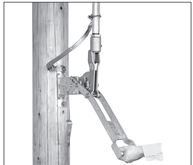
Figure 23. Verifying the stack has been taken up in the operating linkage.
