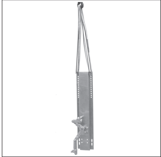
Figure 8. Hoisting the bell-crank into position.
