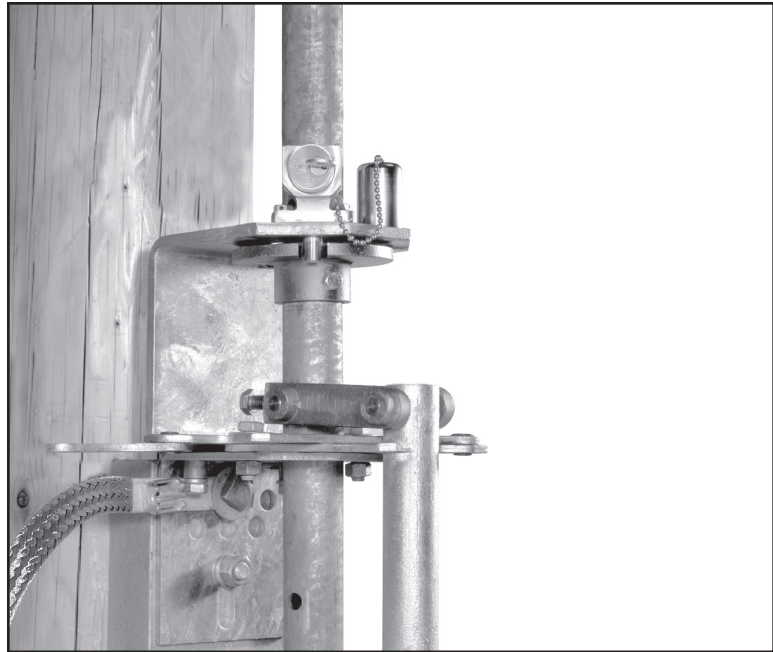
Figure 20. Attach the foot-bearing assembly.
