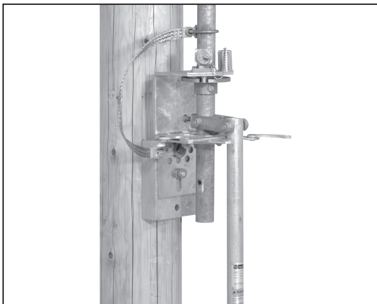
Figure 32. Disengage the key interlock bolt.
