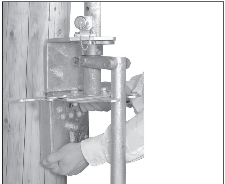
Figure 19. Position the interlock bracket, locking disc, operating handle assembly, and foot-bearing assembly onto the lowest vertical operating pipe section.
