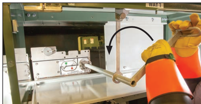
Figure 15. Resetting the fault interrupter after a fault.
