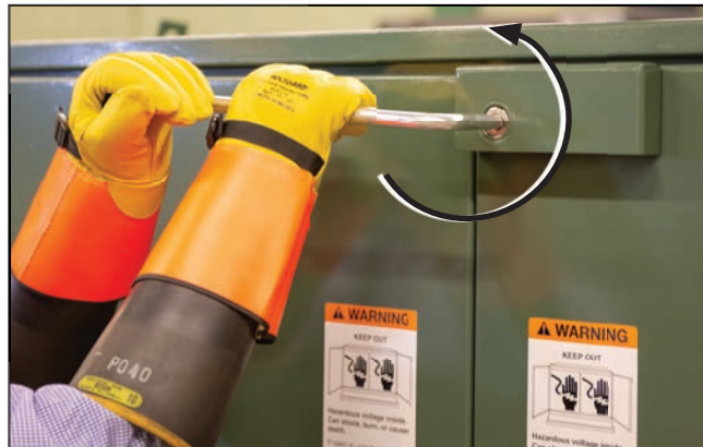
Figure 3. To unlock the front doors, turn the pentahead socket wrench 60° counterclockwise against spring resistance until a "click" is heard and the wrench reaches its stop.
