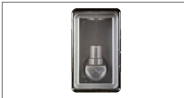
Figure 17. The isolating disconnect after the fault interrupter has been opened and reset.
