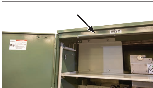
Figure 11. Door holder placed in the storage position to allow the door to close.
