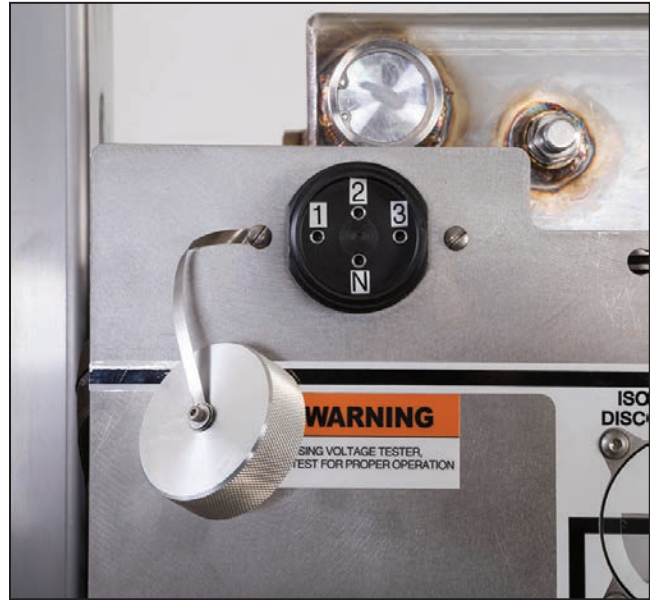
Figure 22. The Potential Indication feature with the cover removed.
