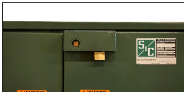
Figure 13. Enclosure doors padlocked.
