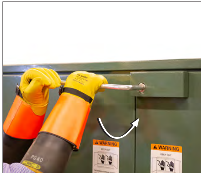
Figure 4. To unlock the front doors, turn the pentahead socket wrench 60° counterclockwise against spring resistance until a “click” is heard and the wrench or tool reaches its stop.
