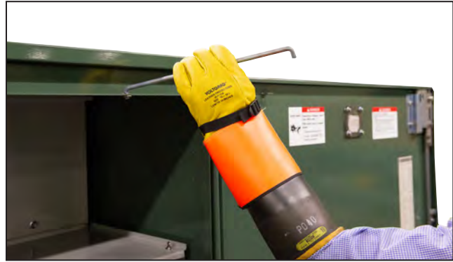
Figure 10. Lift the door holder to allow the door to swing closed.
