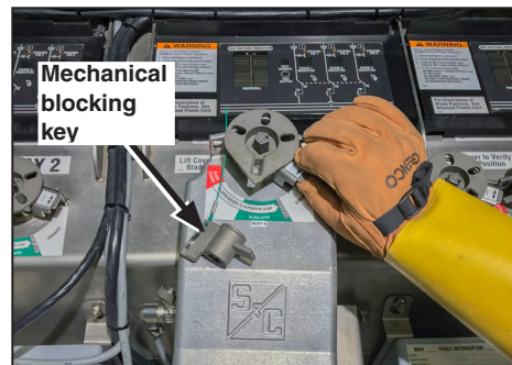
Figure 6. Removing the mechanical blocking key and moving the Operation selector out of the way.
