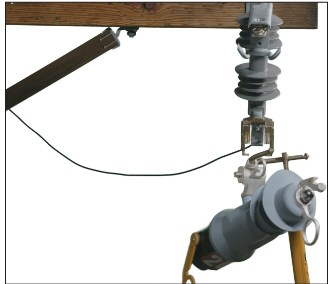
Figure 9. Using a Talon tool during installation.
