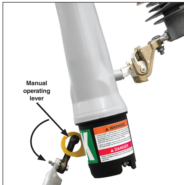
Figure 11. The manual operating lever in the Up position.
