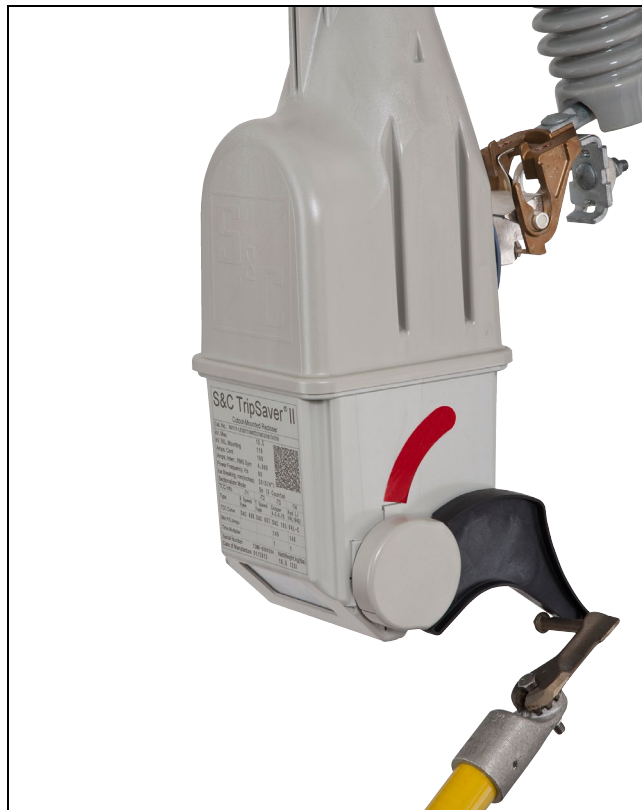
Figure 22. Place the prong under the lever and push it up.
