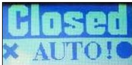
Figure 50. Exclamation point indicator for a battery abnormality.
