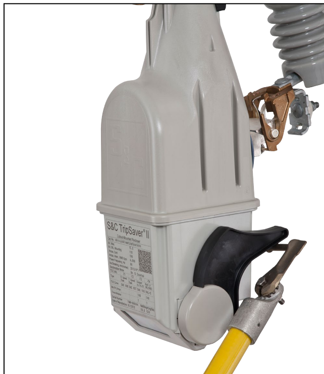
Figure 23. The curved label must be completely covered.
