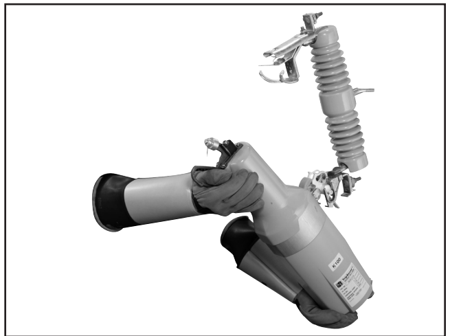
Figure 6b. Inserting 15/27-kV TripSaver Dropout Recloser into mounting.
