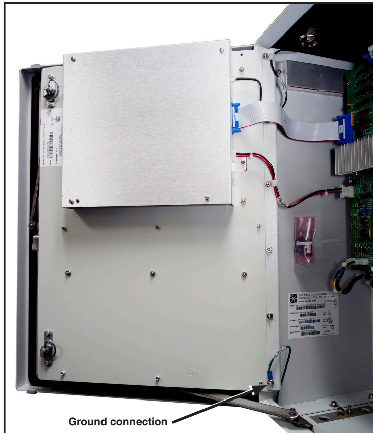
Figure 13. Completed front panel installation, without Communication option plate.
