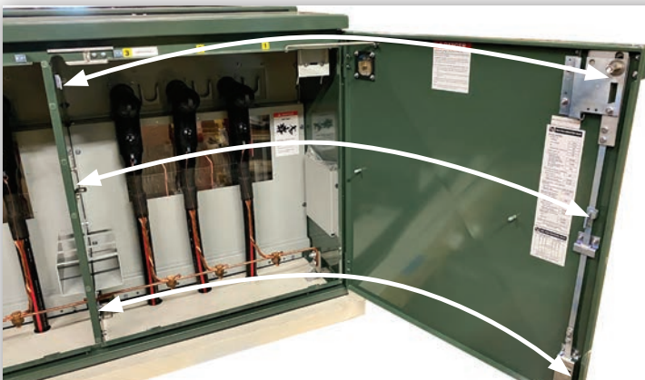
FIGURE 7. Two-step controlled opening of doors.
