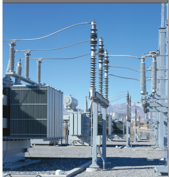
138-kV Trans-Rupter II, Model EX protects step-up transformer.
